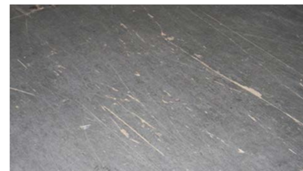
☰ Flooring: Slight deformation, superficial wear
