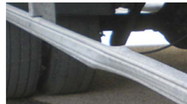
Side underun guards: Deformation beyond economic repair
