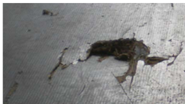
🔧 Flooring: Deformations or perforations within economic repair
