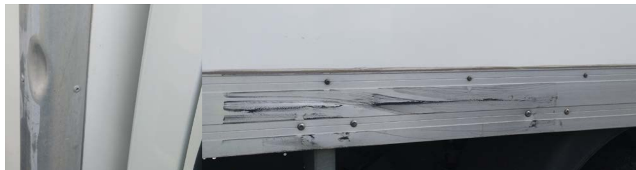
Underbody side profiles: Deformations within economic repair
