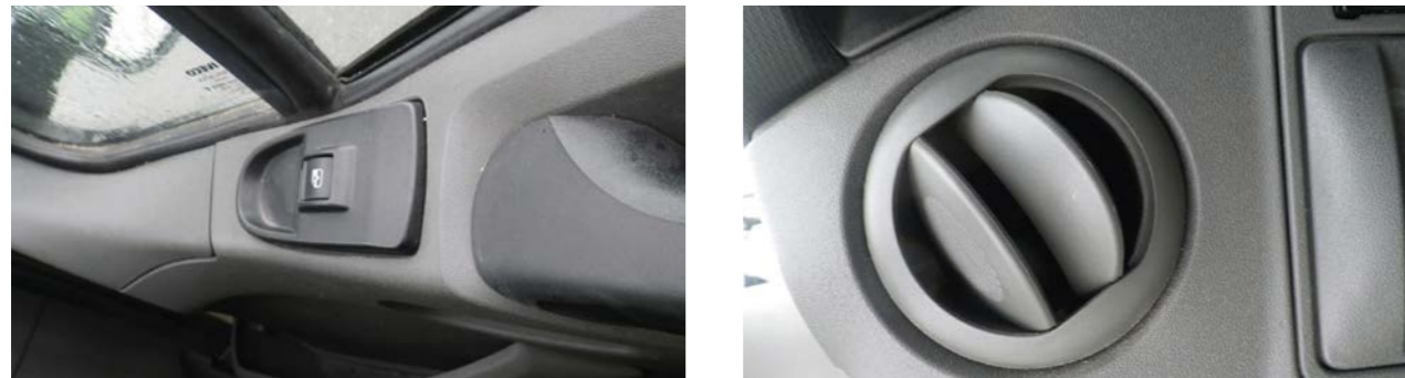
Slight discoloration due to sun exposure
