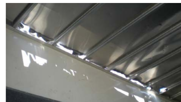
↻ Roof space: Frame damaged, fabric not within economic repair
