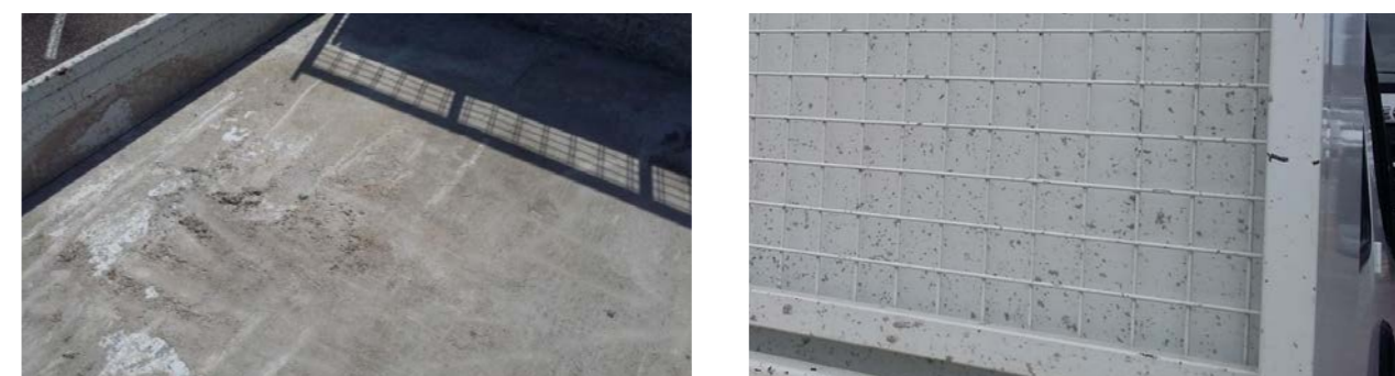
Trace of concrete or chemical product covering \geq 1/4 of the surface of the bed
